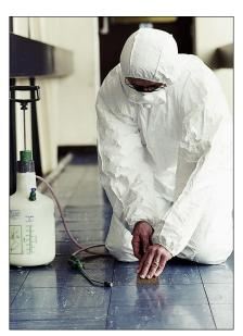
Spray at low pressure; high pressure spray could disturb fibres from asbestos paper under these tiles
